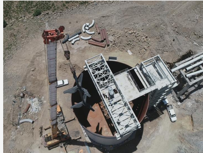
Copper Tailing Holding Tank 200kw, Impeller dia5.9m, Weight:19.5 ton
